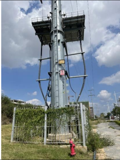
8#塔基植被恢复
