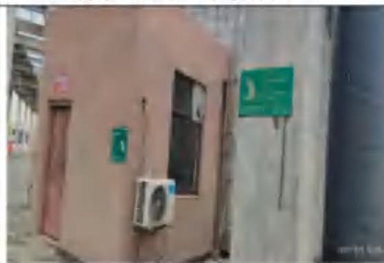
中景石化在线监测房及污水排放口标识
