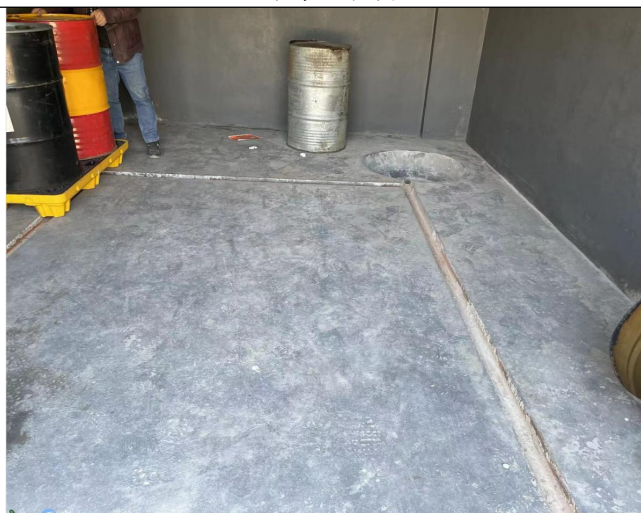
危废贮存区导流沟槽
